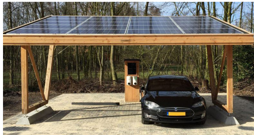
Solar panel trellis
