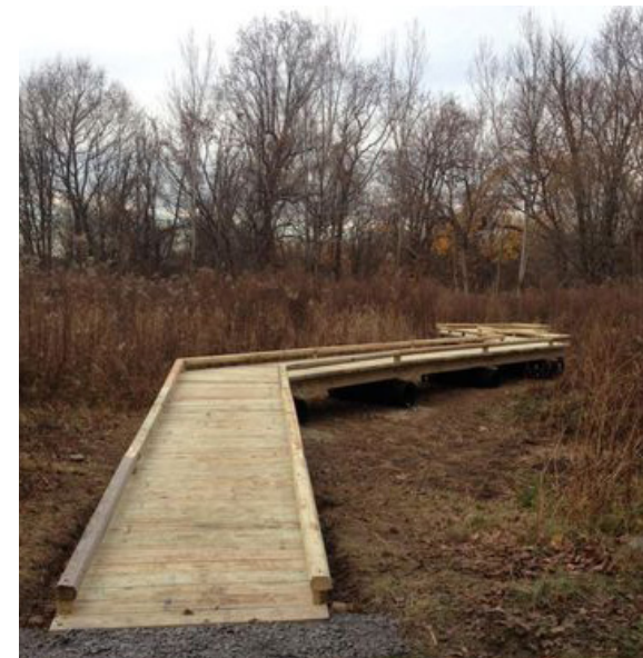
Elevated boardwalk path- great for areas where minimal earth disturbance is required
